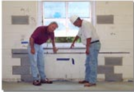
Lesco's Doug Dizney (right) and Jim Hadley of Sika Corporation inspect work.
