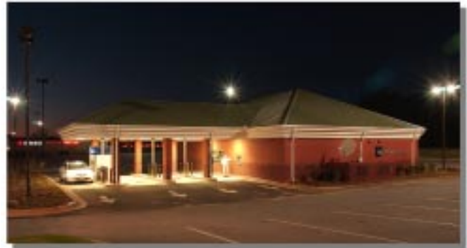
Customer safety is top priority at Wachovia's 3,000 locations from Georgia to Connecticut.
