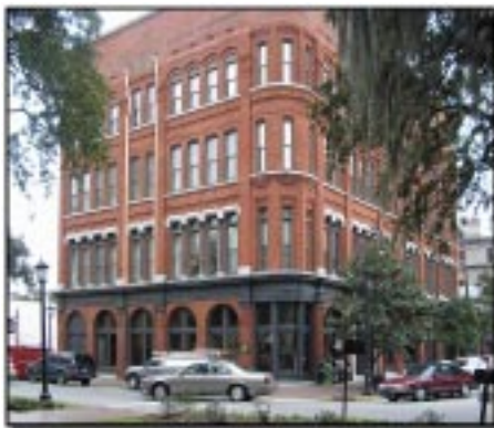
Wachovia's Bull Street location in downtown Savannah received extensive interior and exterior restoration work.
